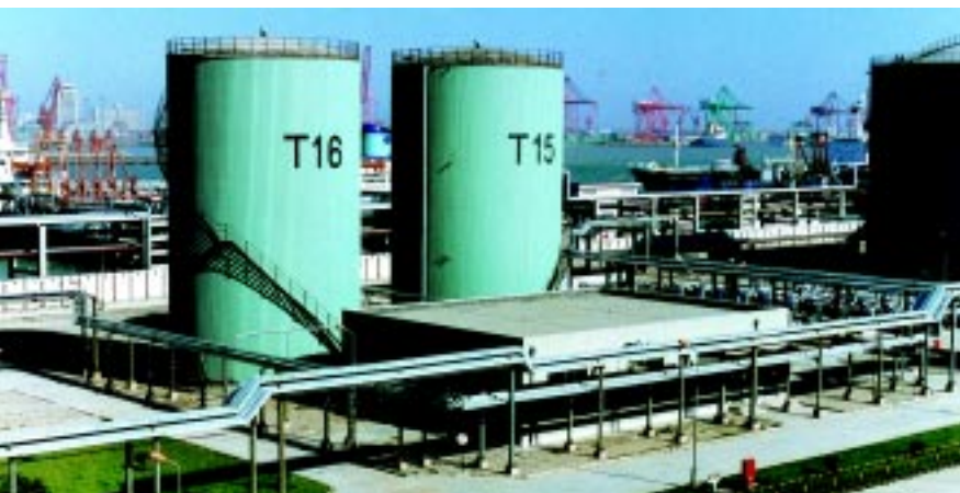
The tank farm of Tianjin International Petroleum Storage and Transportation Companies
