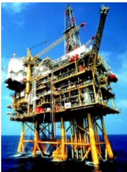
The Xijiang 24-3 oil production platform in the South China Sea
