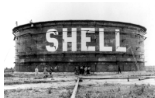
Construction of a storage tank at a Shell installation in Shanghai in the 1930s
